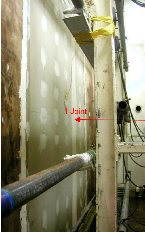
Fig 2: Test specimen surface under-test comes with 1 joint (inside chamber view)
